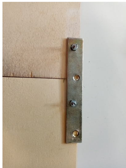
A way to join two plywood panels together if you want the racetrack to be longer.
