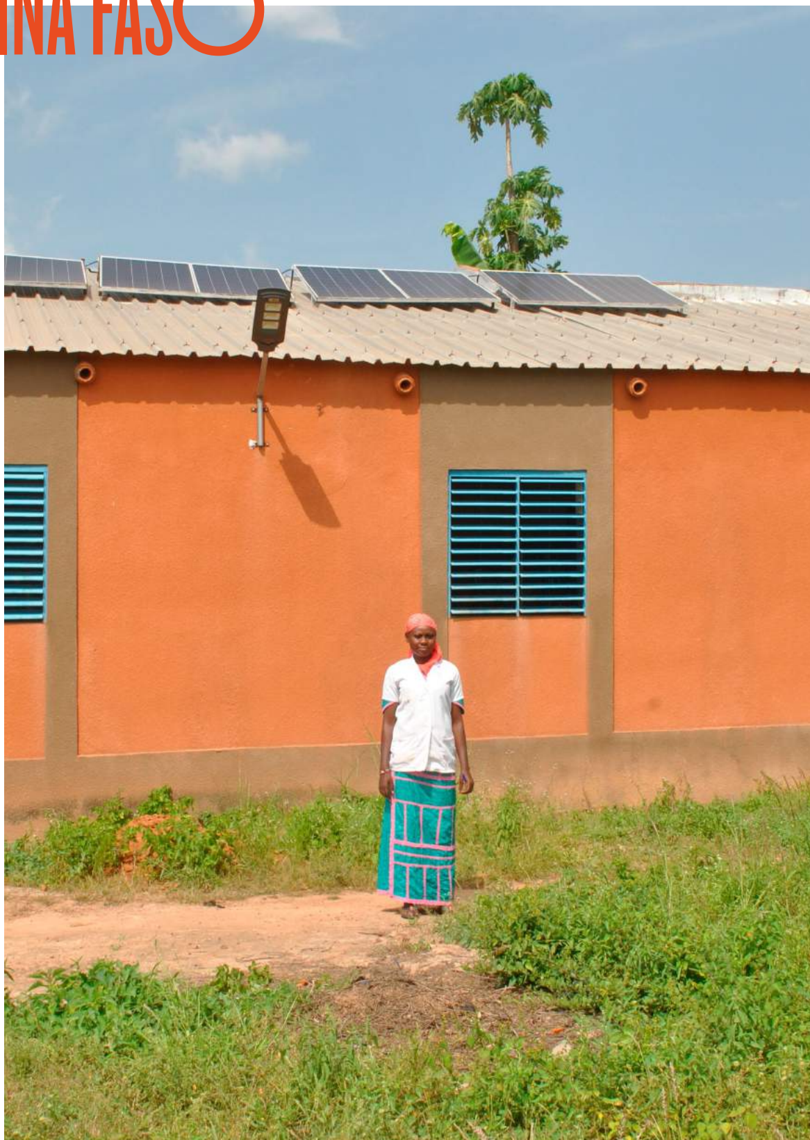
Nurse Kadi Paré in front of her solarised health centre in the village of Tintilou, Burkina Faso.
