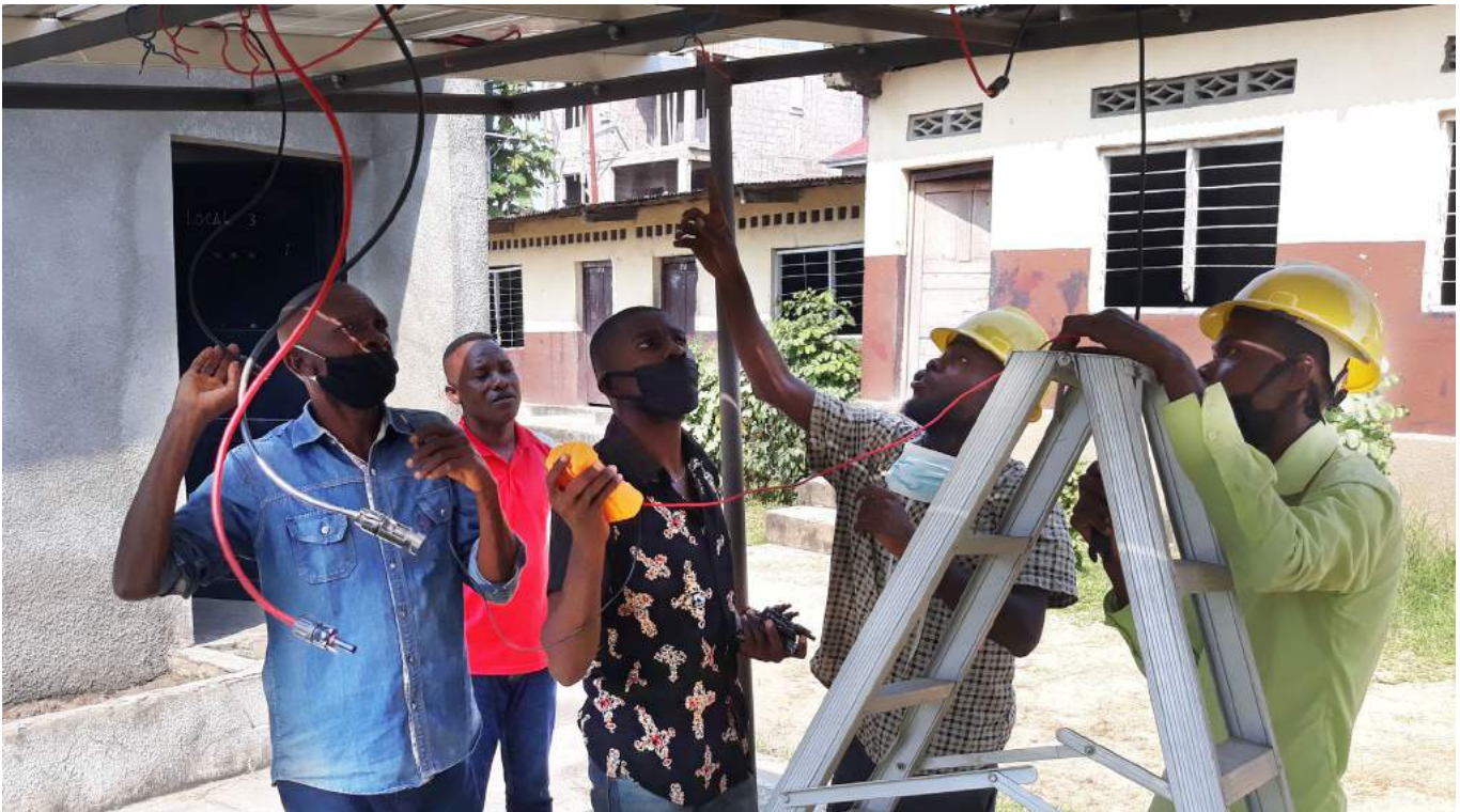
Apprentices and teachers install the in-house solar system at Eproba.
