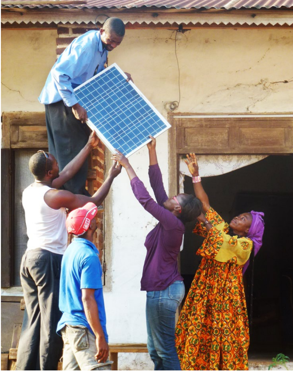
Installation of a solar system in Central Cameroon.
